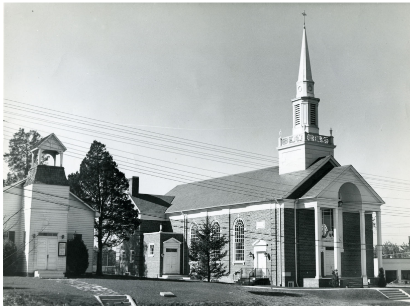
Marvin Memorial United Methodist Church about 1949, showing the original "Little White Chapel" from 1872 at left. The photo was taken from the Woodmoor Shopping Center looking across Old Bladensburg Road, now University Boulevard. Photo Courtesy of Don Messersmith, Silver Spring UMC.
