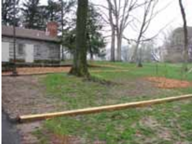
Long pieces of wood were placed along the slope outside the Rec Center to help prevent erosion of the soil.
