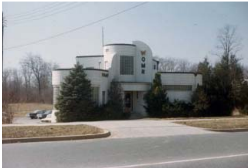
The WQMR radio transmitter on Arcola Avenue in Kemp Mill.
