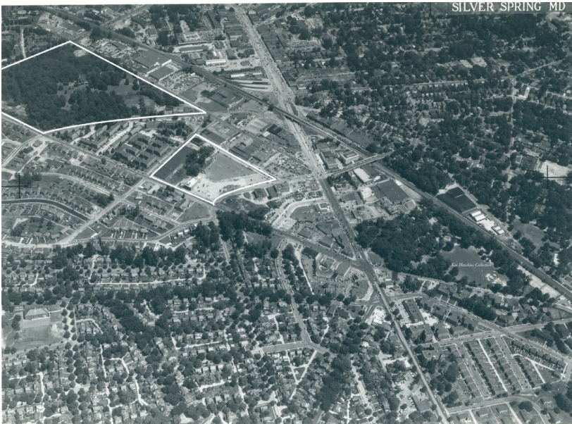
The center of downtown Silver Spring, Maryland, view north and east over Georgia Avenue at the line with the District of Columbia. The remaining Blair estates are outlined in white at the upper left. M. Blair’s house at this location was demolished in 1958 for apartment towers and a small shopping center. The location of his father’s earlier house was near the small triangle of land to the southeast of the parcel shown, which is the location of the old Silver Spring, today’s Acorn Park. Commercial aerial photo circa 1955. Courtesy Ken Hawkins.
