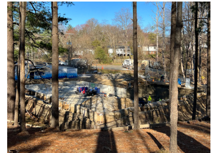
The old pool was removed.
