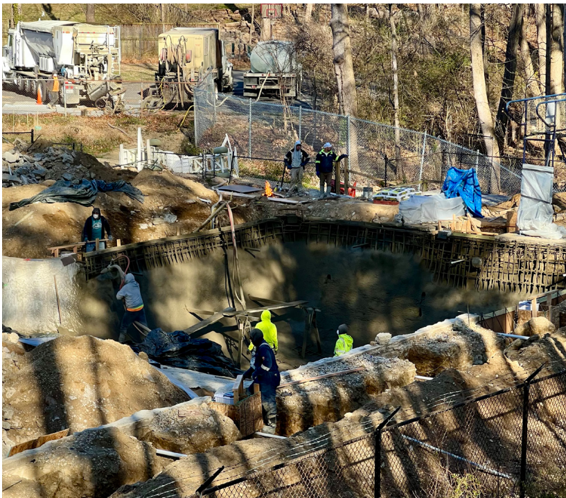
Workers spray concrete onto the framing already put in place around the newly remodeled deep end of Forest Knolls Pool. The pool is expected to reopen at the end of May as usual.
